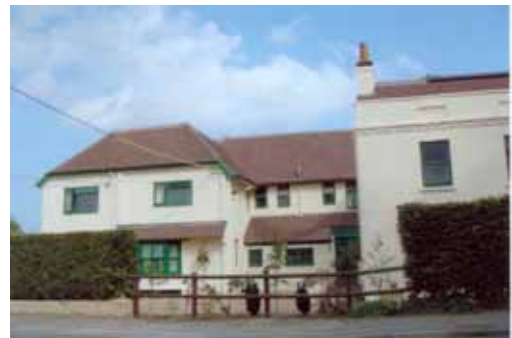
Elderfield after renovation
